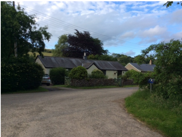
Viewpoint G – view of applicant dwelling + adjacent property, full extent of extension will be unread from this aspect
